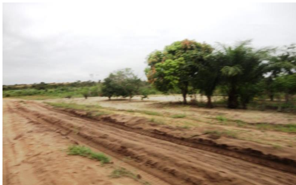
Photo 2: beginning of aggravation of the ruts at the entrance of the village Loumou
