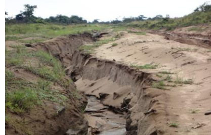
Photo 5: : Evolved rut in longitudinal gully at the exit of Case Barnier
