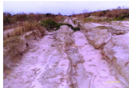
Photo 3 : Evolved ruts in linear channels to Ntoba Ilélé
