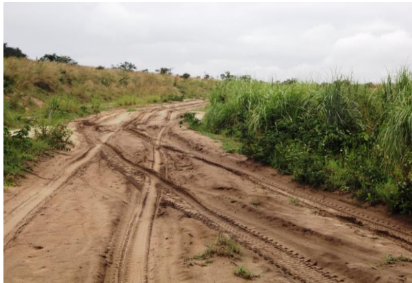
Photo 1: trace of wheels and beginning of rutting in the area of Loumou schools
